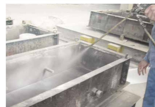
Spray-coating of a mould
