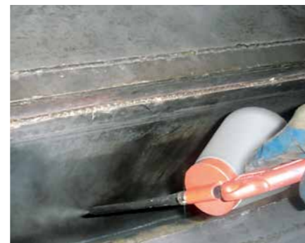
Surface spray coating of slab mould
