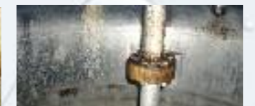
Cleaned tanks after full automatic cleaning procedure.
