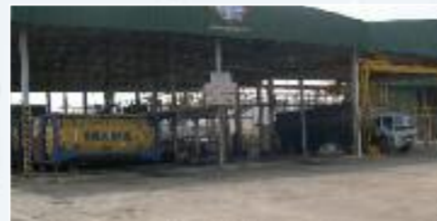
Tank cleaning station in Asia region for tank trucks and containers.
